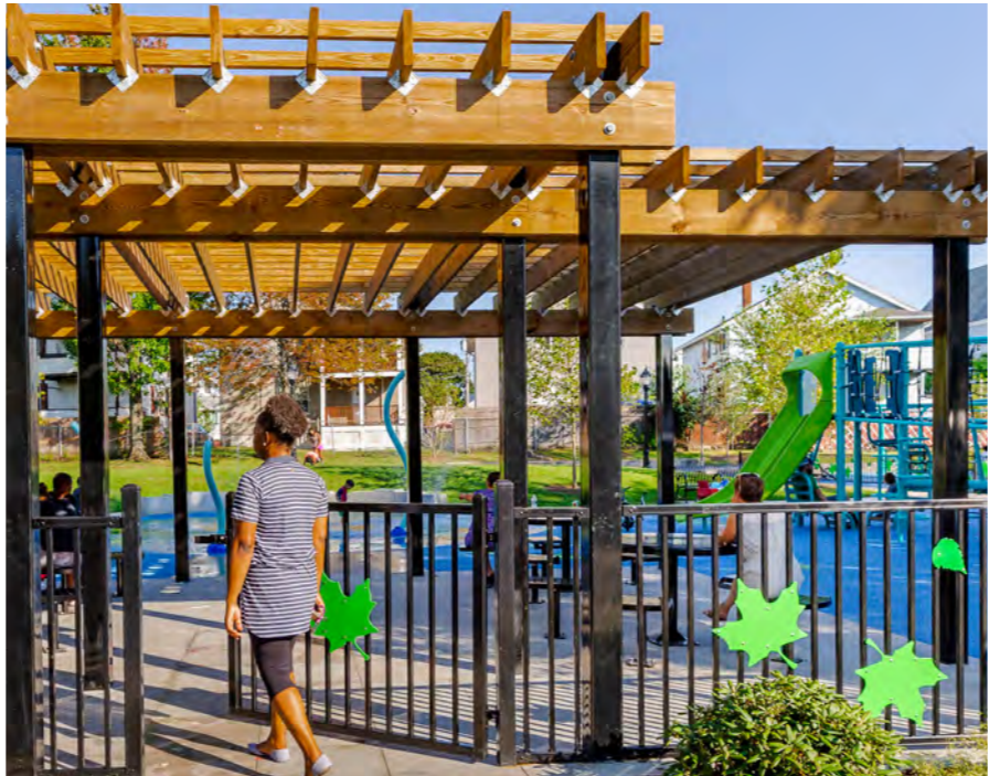
Fencing and Shade Structures Gramstorff Park - Everett
